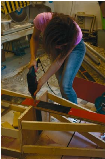
Figure 12. Frame of the formwork
