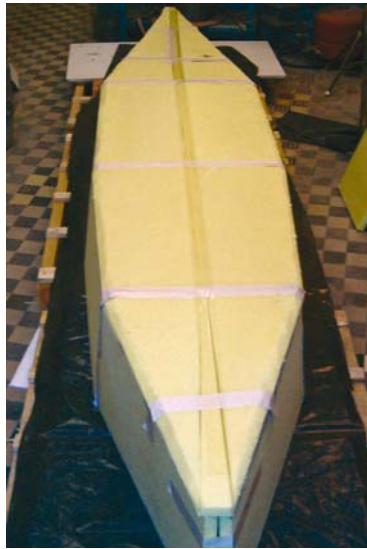
Figure 13. Extruded polystyrene formwork
