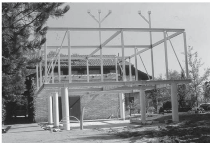
Figure 12. Picture of the structure during construction.
