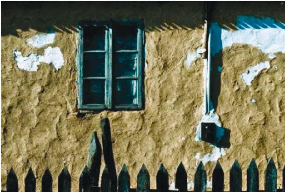
Fig.2. Detail of an earthen building
