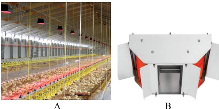
Figure 1. Radiating units placed on the roof (A), heating unit (B) that uses gas- or electric energy [12]
