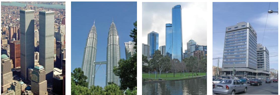
Figure 14. Twin high-rise towers: the former WTC in N.Y.C., the Petronas in Kuala Lumpur, Melbourne's Rialto and the Hermina Towers in Budapest
