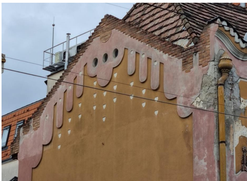
Photo 12. The secondary façade from the Bartók Béla street' view.
