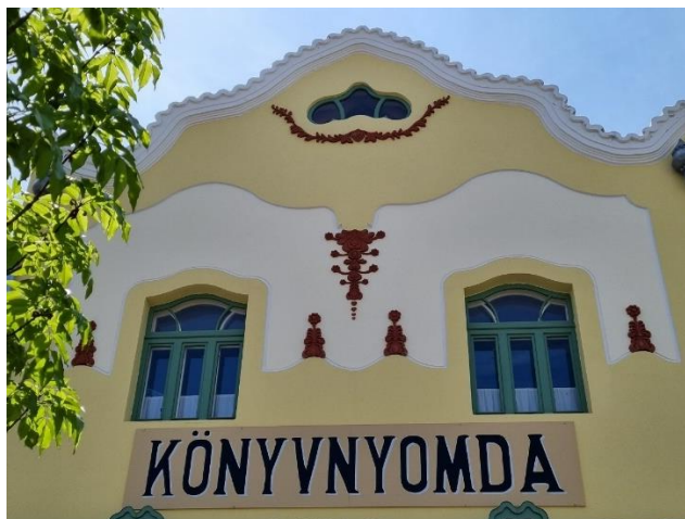
Photo 16. The original-coloured decoration
