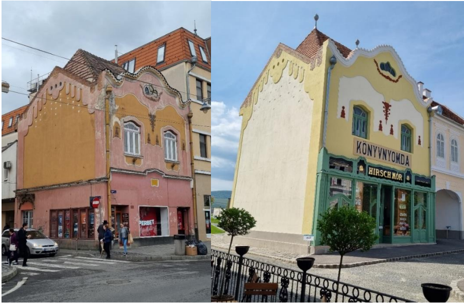
Photo 6. The original building found in Târgu-Mureș - comparison Photo 7. The building replica found in Szentendre Museum
