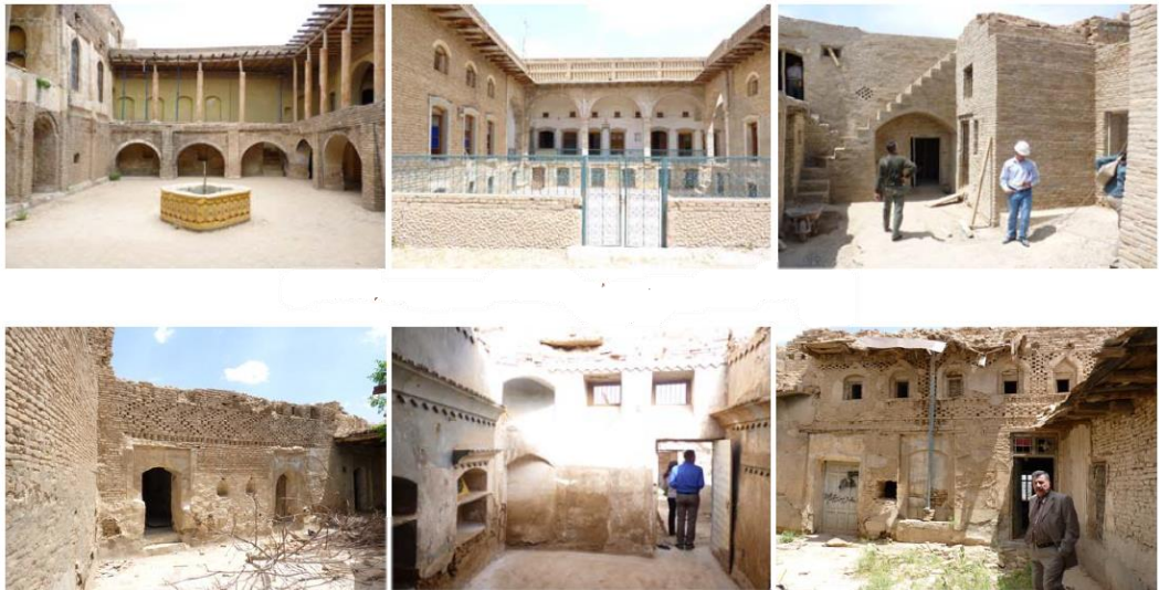
Figure 3: Erbil Citadel Houses renovations work. Reference: [4]
